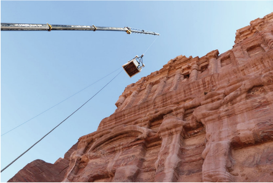
Fig. 3 Survey mission of international experts to evaluate the conservation status of the Palace Tomb and assess priority of interventions, including rehabilitation of the water channel and cleaning of cisterns carried out by workers from the local communities. Photo Alessandra Blasi
