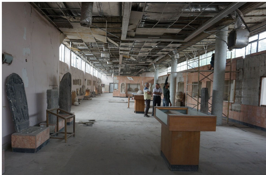
Fig. 5 June 2023. Post-earthquake damage assessment on the first floor of the museum building with ReStruere and Unifi team. © Aleppo project
