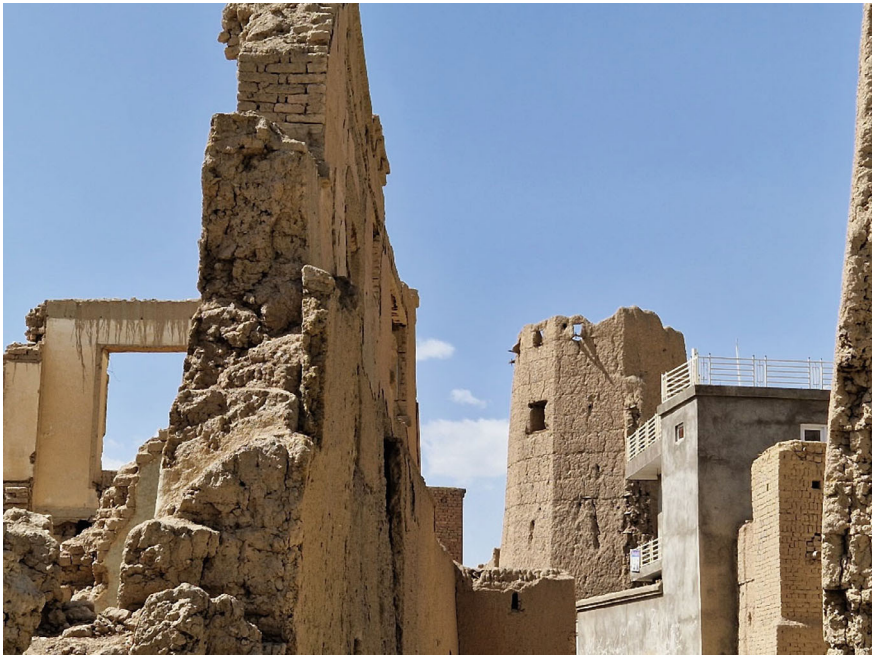
Fig. 4 Concrete interventions in a qal'a in Tolwara ( Photo M. Loda 2023)
