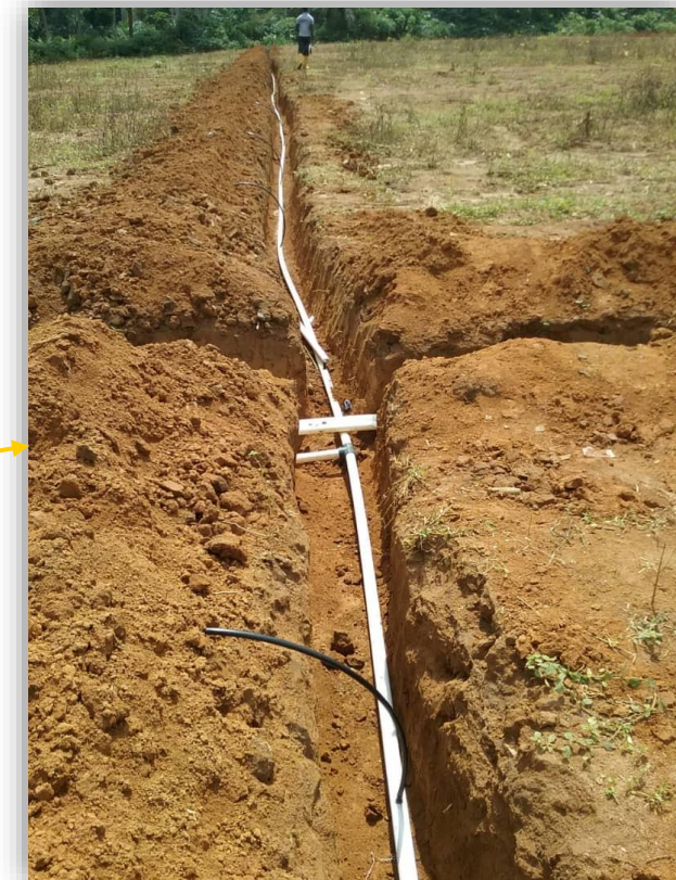
Main underground canalisation system
